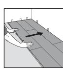
9. After 2-3 rows. Adjust the distance to the front wall by leaving an expansion gap of 3/8" (10mm).
