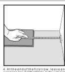
4. At the end of the firstrow, leave an expansion gap of 3/8" (10mm), to the wall and measure the length of the last plank to fit.
